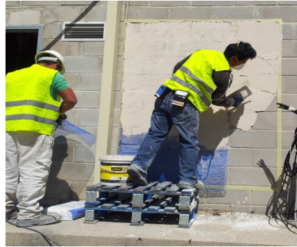
Application of depollutant mortar (nanoTiO 2 )
