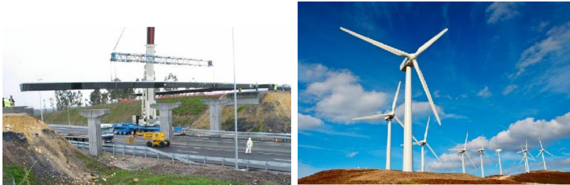
Figure 4.46 m long carbon fiber pre-preg primary beams for a road bridge in Spain (left) and a composite wind turbine beam (right).
