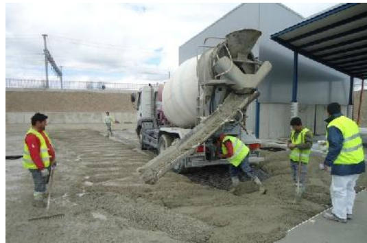
Figure 23. In situ preparation, mixing and application of photocatalytic concrete in a bus station in Ávila, Spain
