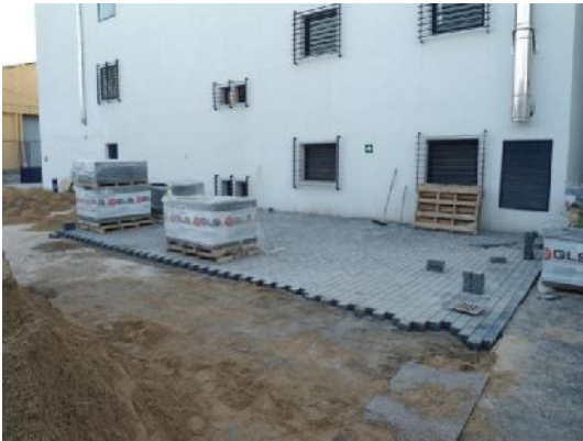
Figure 22. Assembly of paving stones at ACCIONA's parking lots in Madrid
