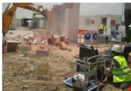
Figure 8. Monitoring point – Operator (worker 2)
