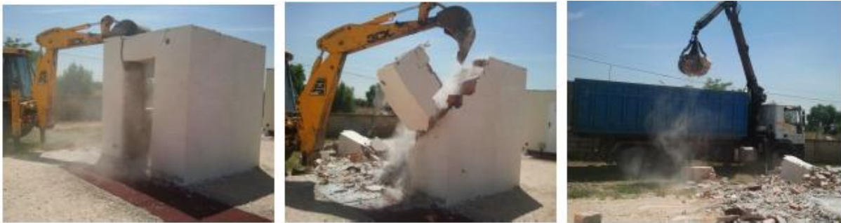
Figure 7. Snapshots of the cabins demolition (left & middle) and waste collection (right).
