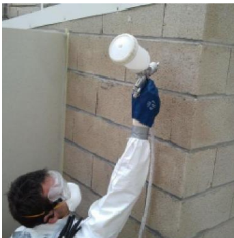
Figure 1. Application of self-cleaning coating on a vertical wall.
