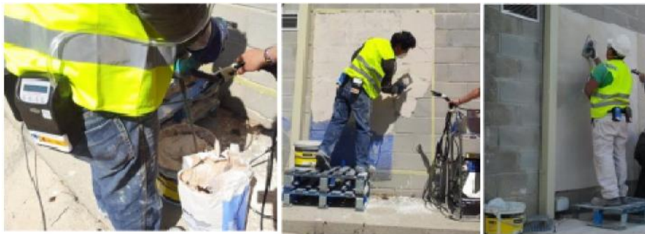
Figure 6. Snapshots of the process; Mixing (left), Application (middle) and Scrapping (right).
