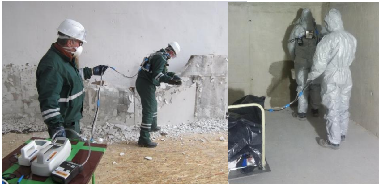
Figure 4: Workers in Romania and Poland performing various works involving materials with MNMs, with simultaneous measurement of the NP concentrations in air.
