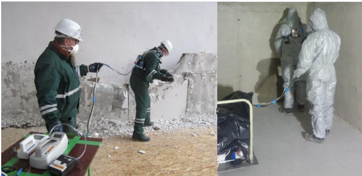
Figure 2: Workers in Romania and Poland performing various works involving materials with MNMs, with simultaneous measurement of the NP concentrations in air.
